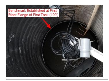
Establish benchmark at the flange in the first riser of the first septic tank, as shown here.
